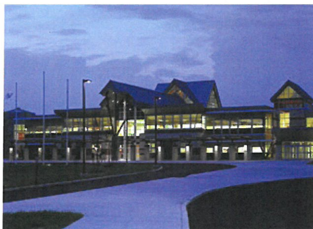
New Central York High School York, PA
