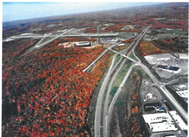
Johnstown Galleria Interchange Johnstown, PA
