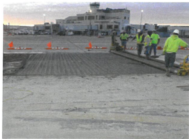
Central West Virginia Regional Airport Authority Taxiway Rehabilitation Yeager Airport, Charleston, WV
