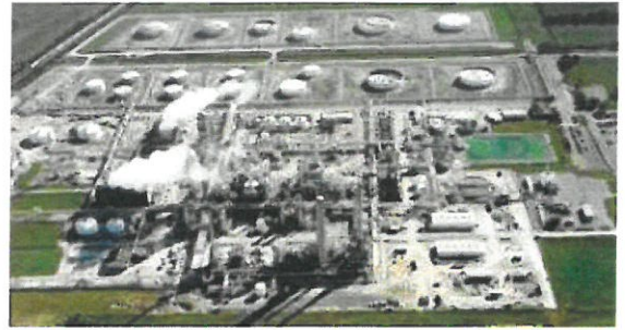
COSMAR Modernization Project Carville, LA
